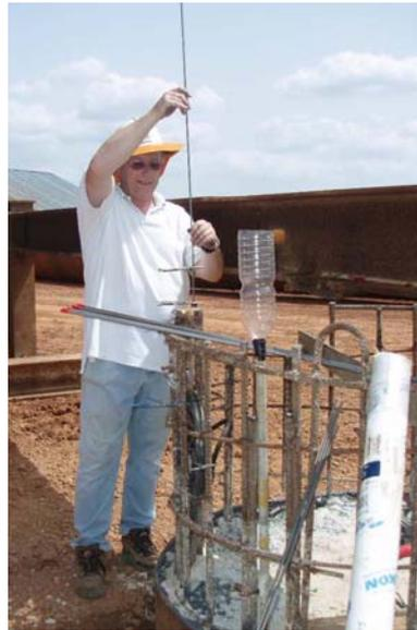
If not previously installed, the telltale rods (6 or 8mm) need to be coupled together and inserted so that movement of the top of the upper bearing plate can be monitored. Upward movement of the element of the pile above the O-cell is typically determined by measuring the compression between the top of the O-cell assembly and the top of the pile and adding this to the upward movement of the pile.
