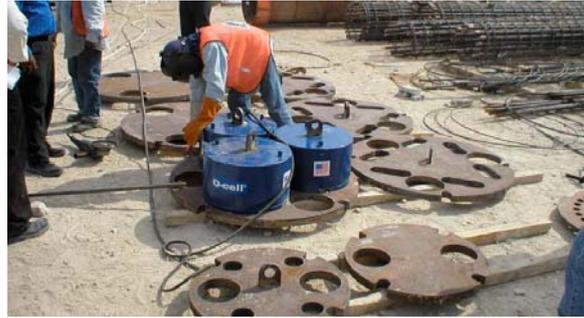
The O-cell(s) are accurately positioned on the lower bearing plate and welded into place. Temporary lifting eyes are often used to facilitate handling of the plates and O-cell(s).
