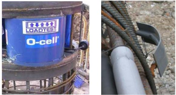
A suitable number of spacers/rollers/skids should be used to ensure that the reinforcing cage remains central to the bore as the cage is lowered.
