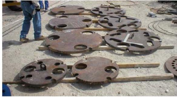
The bearing plates, fabricated locally, are designed specifically for the reinforcing cage and number of O-cell(s) required for the desired load to be mobilised in the test pile.
