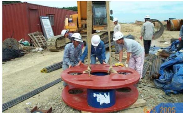
Once the bottom plate and O-cell(s) are secured, the top bearing plate is accurately aligned and welded into place. Three or four vertical bars are also welded between the plates to prevent any torsional forces being transmitted to the O-cell(s) during handling.
