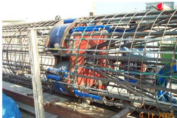
Traditional telltale casing and rod extensometers extending from the top of the O-cell assembly to top of pile and any ECTs, used to measure the pile compression can be installed. Hydraulic hoses, can be connected to the O-cell assembly and routed through the reinforcement.
