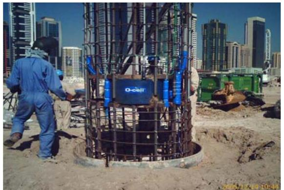
The temporary stiffening bars between the bearing plates (for handling purposes) will be cut just above the bottom plate. Top of the bottom bearing plate will be greased to aid development of the fracture plane at this level.
