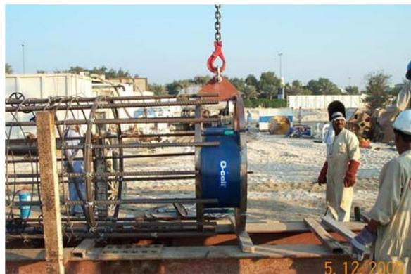
The completed O-cell assembly will then be lifted into one side of the reinforcing cage and welded once in the correct position, perpendicular to the cage axis at the given location. Depending on the configuration, sometimes the bearing plates are butt welded to the cage(s).
