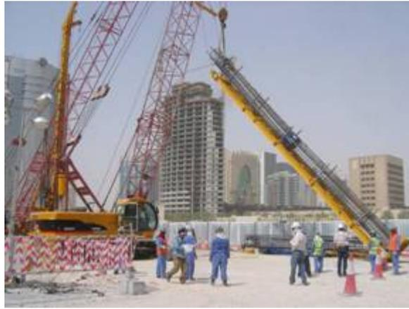
The lifting of each cage to vertical should be carried out using a lifting beam or several pick points to ensure the cage remains reasonably straight during lifting.
