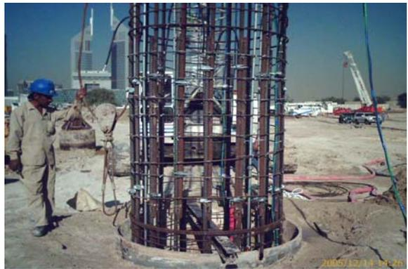
Where cage splices are required, all of the cables from the instruments of the lower cage need to be pulled up to the top of the additional cage and secured in place.
