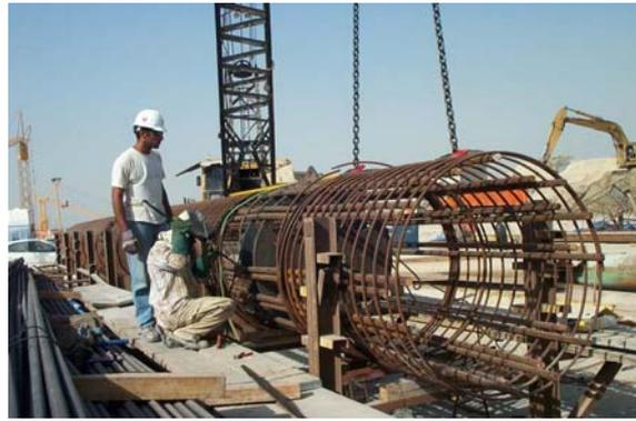
The cage for the other side of the O-cell assembly can then be positioned and welded as required. The funnel to guide the tremie passed the O-cell level can be constructed. Assembly of the cage on a flat surface is advisable.
