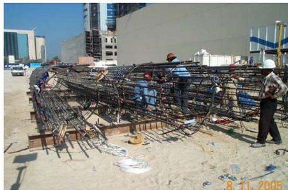
Any additional cages that will be spliced together over the bore need to be prepared – installing lengths of hydraulic hoses and telltale and vent casing extensions with union couplers for rapid connection and any strain gauges required.
