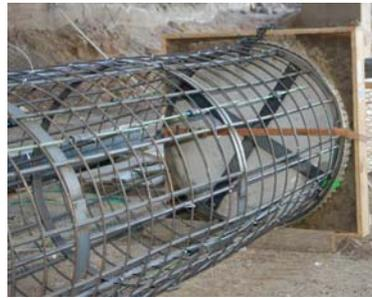
Once the welding of the O-cell cage is complete the instrumentation can be fixed. LVWDTs across the bearing plates, strain gauges, rod extensometers and telltale casing will be attached to the cage. Where specified, pressure sensors or pile tip pressure plates can be fitted. All cables are routed and secured along the reinforcing cage and temporarily fixed inside the top of the cage.
